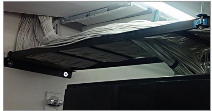
*Figure 4:* A switch closet of a small company. The left side picture shows the main switch rack with huge bundles of cables intertwined with each other. The right side picture shows the huge bundle of cables going to riser channels and lateral ceilings from the rack.
