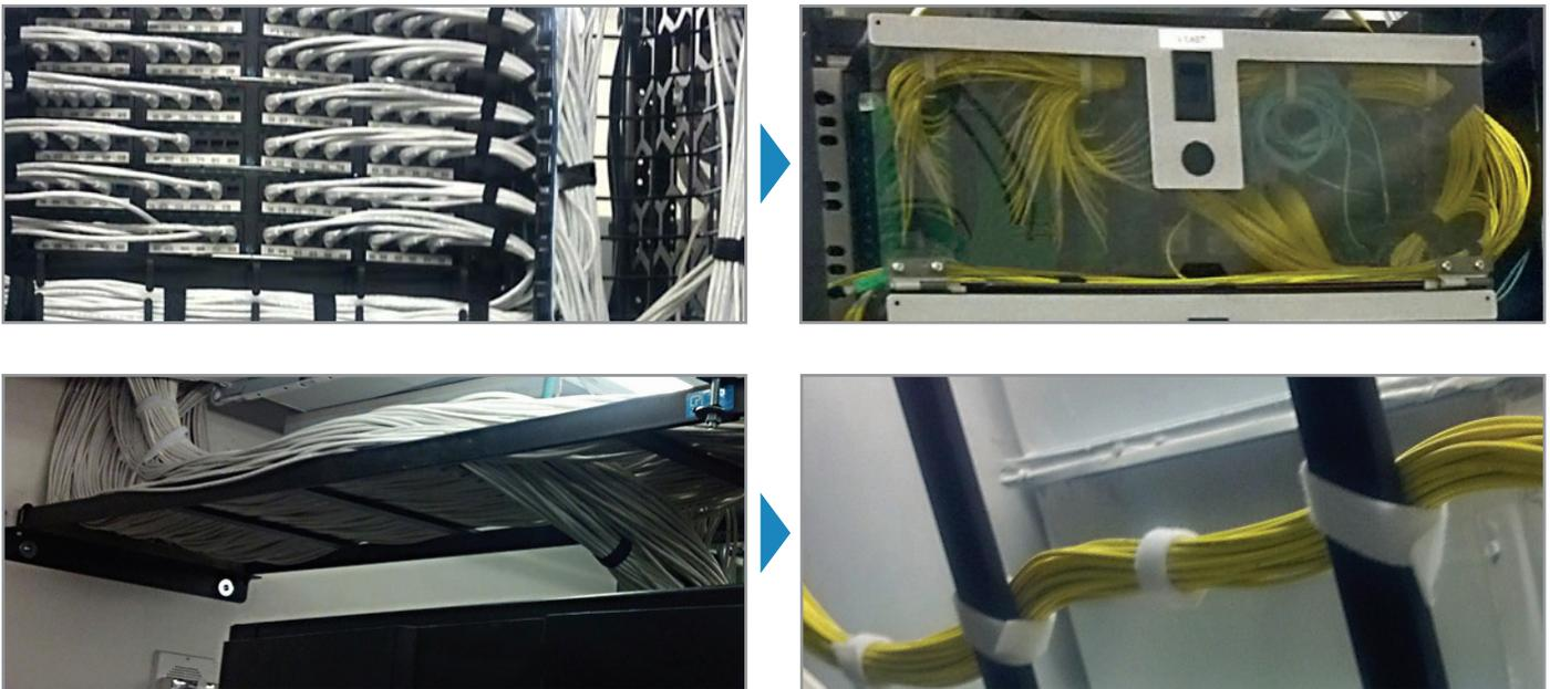
*Figure 7:* Cable size of CAT 5 vs. optical fiber Implemented in the same building infrastructure. The rack and cables at the left side were an early LAN implementation supporting one half floor. The yellow cables at the right side are the Passive Optical LAN implementation to replace the original LAN implementation — supporting three and one half floors.
